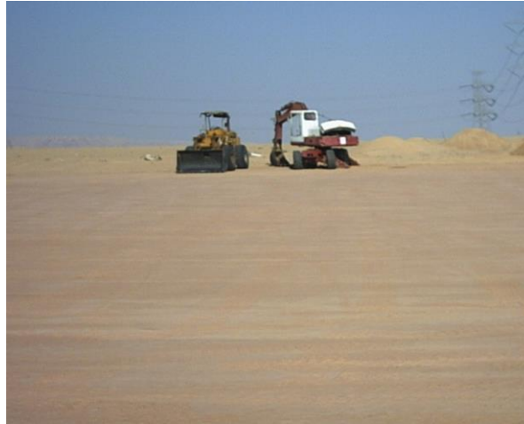
Area Preparation for Site Camp
