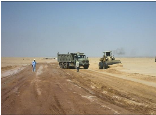
Preparation for Backfilling
