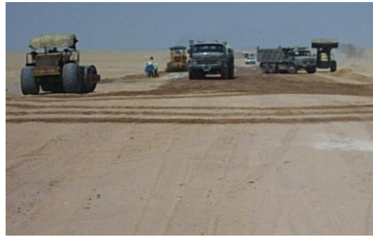
Preparation for Backfilling
