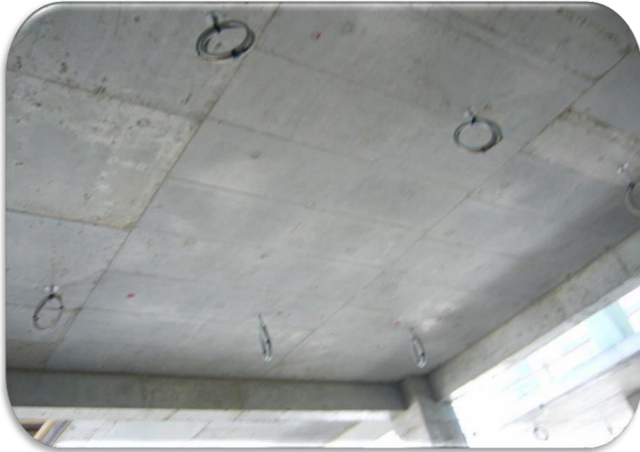
Wires with Flexible Conduits
