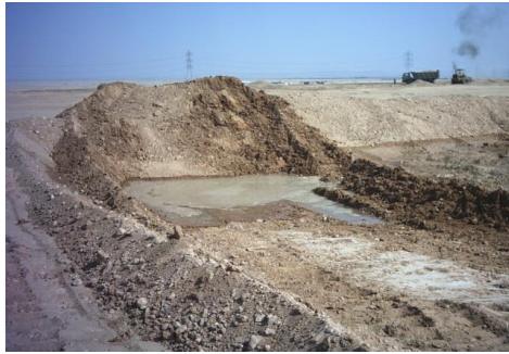
Water Mixing for Back Filling Material
