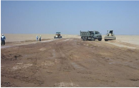
Site Clearing & Preparation for Backfilling
