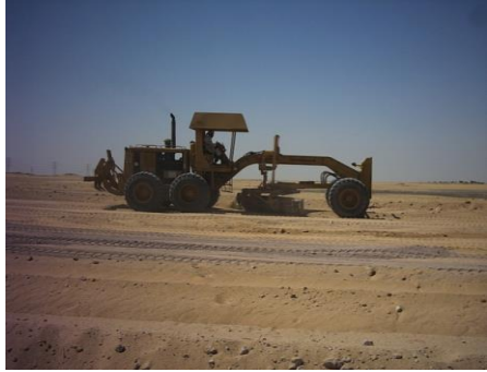
Site Clearing & Grading
