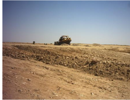
Cutting to Required Levels
