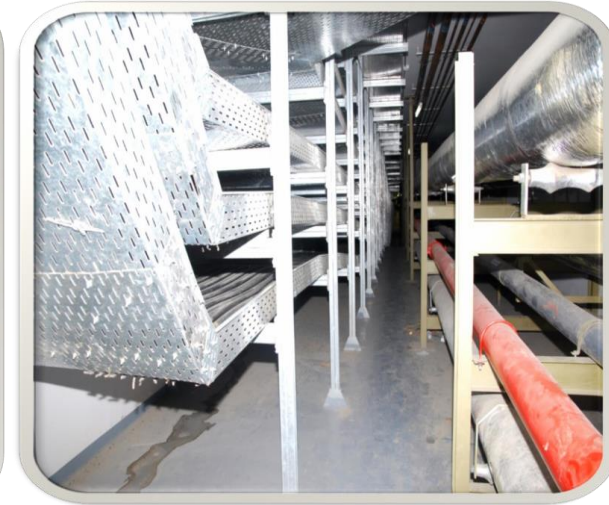
Cable Tray, Round Duct, and Chilled Water Piping Installation
