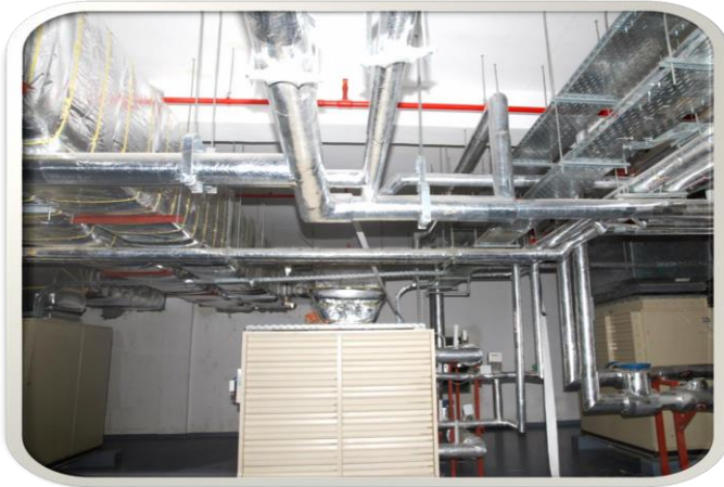
Fixing Ducts, chilled water pipes, and AHUs
