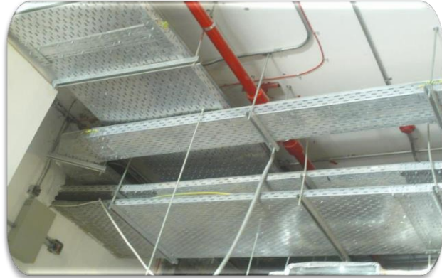
Cable Tray Installation
