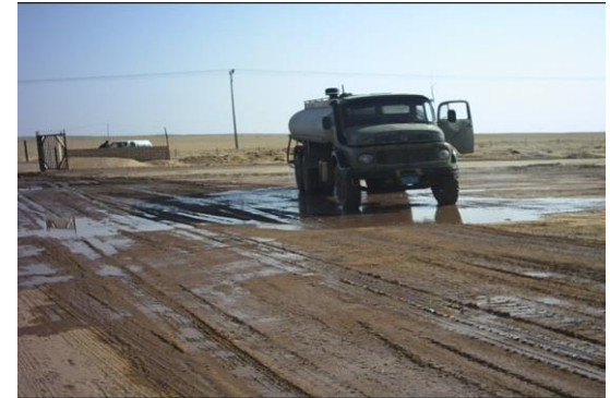
Water spreading prior to Backfilling
