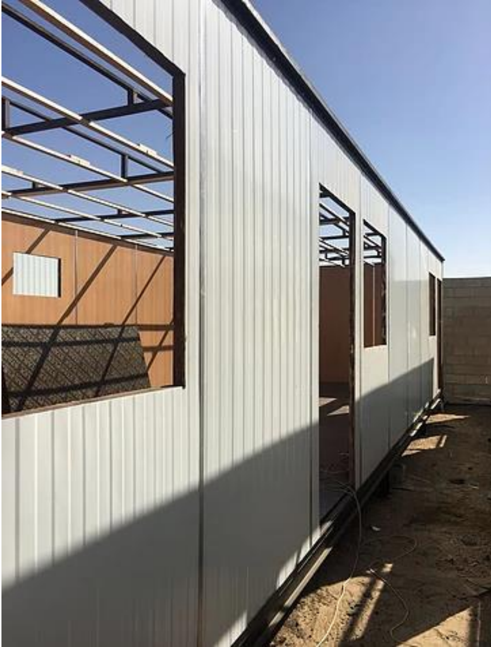
Exterior of portable cabin
